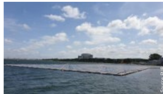
The 1.5MWp floating solar PV systems at Bedok Reservoir and Lower Seletar reservoir collectively generates enough energy to power 800 four-room HDB flats annually
