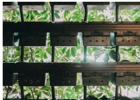
Example of a tray system green wall
