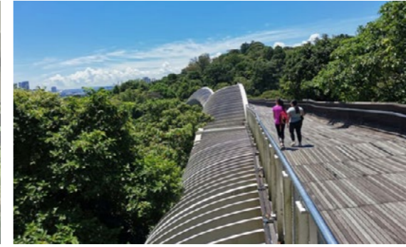
High level bridge connection: Henderson Waves
