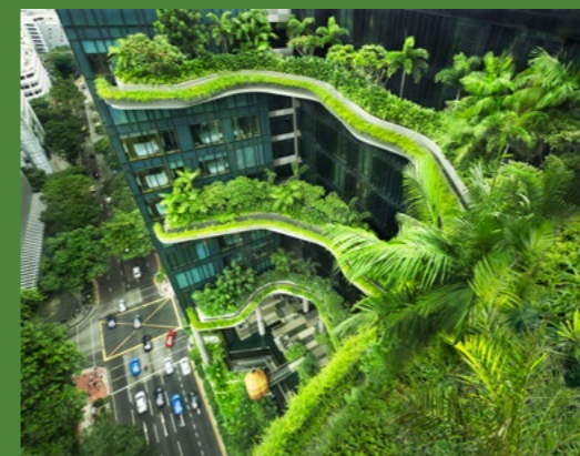
Publicly accessible Communal Planters at PARKROYAL Collection Pickering
