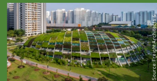
Extensive green roof at Skool4Kidz Campus@Fernvale
